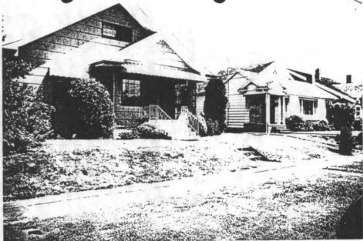
202 3 128 W. 19TH S. FACADE, S. CAPITOL NEIGHBORHOOD H.D., # 39
